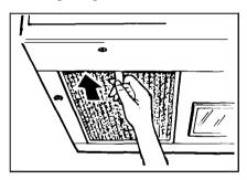
Pull filter upward and to the front to lock into place.
