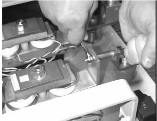
Figure 15. Disconnecting the SCR load side..
