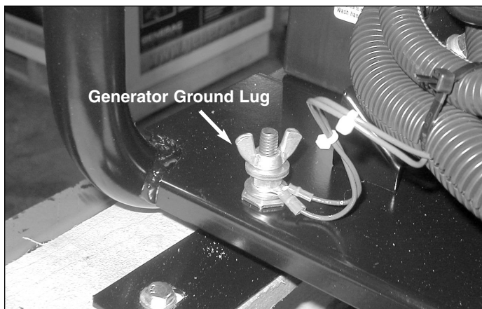
Figure 13 - Grounding the Generator
