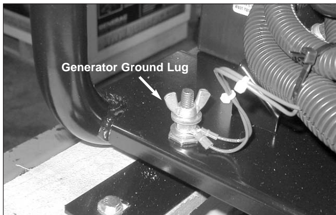
Figure 13 - Grounding the Generator
