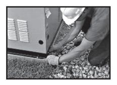
Connect an approved ground strap to the grounding lug on the base frame and to an approved earth ground or grounding rod as specified by local regulations.
