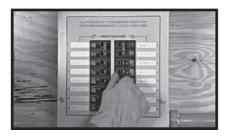
Make sure utility power is OFF and place all of the emergency circuit breakers, in the transfer switch, in the OFF position.
