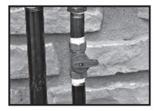
Most applications will require a manual shutoff valve on the fuel line.
