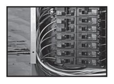
Each wire in the pre-wired transfer switch is color-coded so you can easily match circuits in the main panel to their new breakers in the transfer switch.
