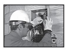
Check to be sure that voltage and frequency from the generator is correct. If line-to-line voltage is not 240 volts, refer to the Installation Guide for the proper adjustment procedures. If line-to-neutral voltage is not 120 volts, check the neutral connection between the generator and transfer switch
