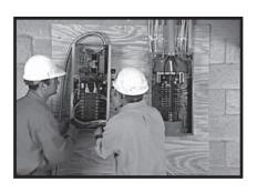
Protect against impact and mount the switch vertically to a rigid support structure. Make sure the switch is level and plumb.
