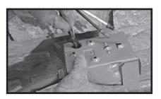
Remove the knockout in the back of the connection box, feed the wires through the back of the box and secure the conduit with the lock nut.
