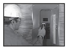
Make sure the 2-pole circuit breaker you installed in the main distribution panel is in the OFF position.
