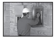
If everything worked properly, switch the main breaker to ON and make sure that power is automatically transferred back to the utility.
