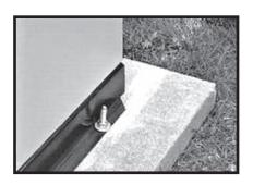
Some locations require the use of a poured concrete mounting pad. If you're using a concrete pad, secure the base frame of the generator to the pad with appropriately sized masonry bolts or other fasteners specified by local code
