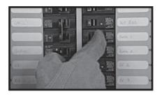
After the engine has completed its cool down cycle and shut down, shut OFF utility power again.
