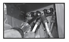
Mount the connection box so that it completely covers the hole in the wall.
