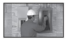
Switch the main breaker ON to restore utility power.
