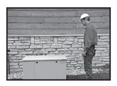
Shut OFF utility power and make sure the generator starts automatically.
