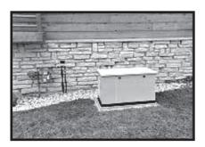
Locate the mounting pad as close as possible to the transfer switch and fuel supply.
