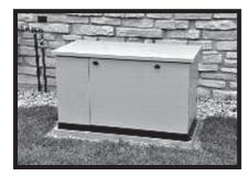
Set the generator onto the pad so that the gravel bed extends several inches beyond the generator on all sides.
