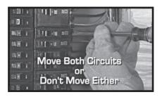
When three-conductor wiring is used, two 120 volt circuits will often share the same neutral wire. To avoid overloading the neutral, you should either move BOTH of the circuits that share the neutral or don't move either of them.
