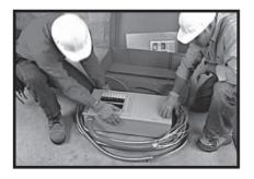
Always inspect the switch for shipping damage. Never mount a transfer switch that shows any evidence of damage.
