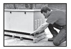
Inspect the generator for shipping damage and, if necessary, file a claim with the shipper.
