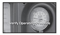
With the generator carrying the entire emergency load, re-check gas pressure to verify that it is at the same level it was before you started the generator.
