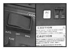
Put the generator's mode switch in MANUAL to start the engine.
