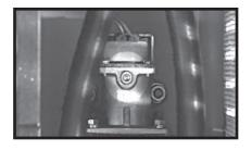
Unhook the gas meter and reinstall the port plug on the regulator.
