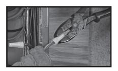
Select a circuit you want to back up and remove the power lead from the breaker. Using UL Listed wire nuts, reconnect the power lead to a matching breaker in the transfer switch
