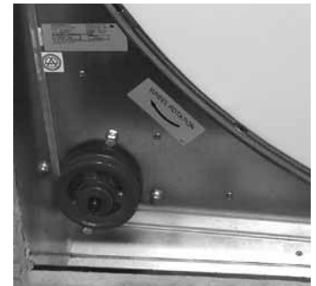
Wheel Belt & Pulley
