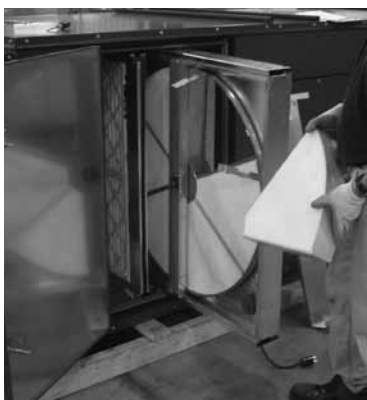
Wheel segment removed
