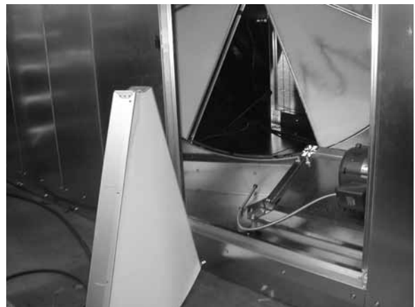
FIGURE 29: Wheel segment removed to allow for cleaning.
