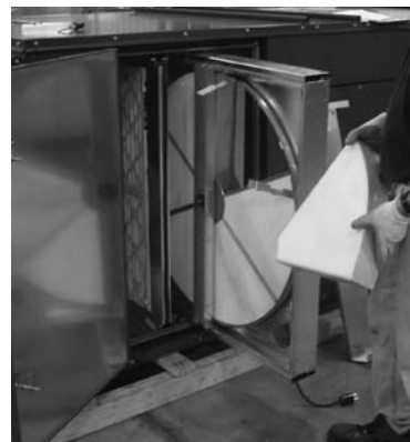
Wheel segment removed
