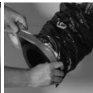
figure 6.4 Finish by taping the duct on the collar.
