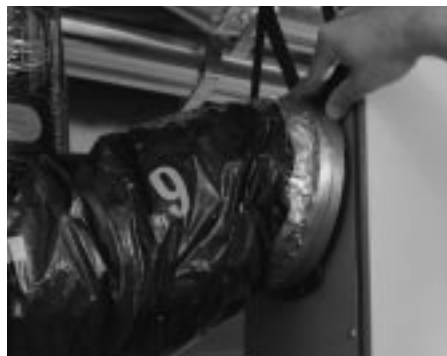
figure 6.5 Slide collar on the unit.
