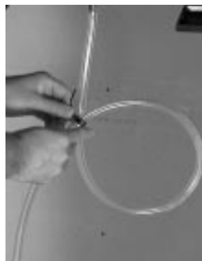
figure 9.3 Make a loop in condensate line
