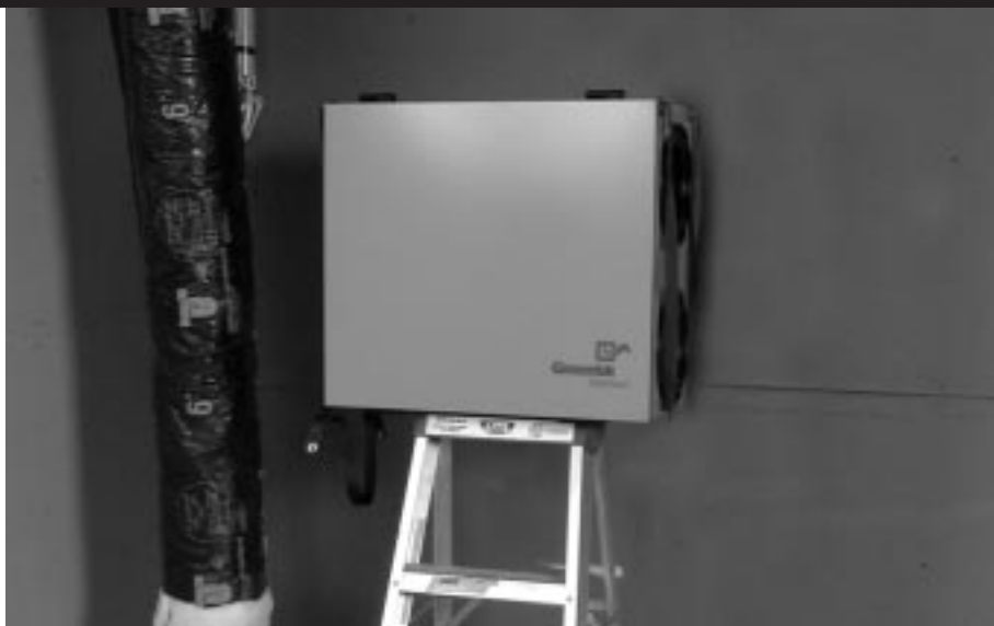
figure 5.1 Place HRV on a stepladder
