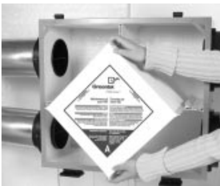
figure 14.3 Slide out the Energy Core
