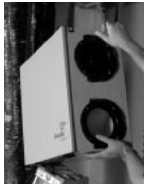
figure 5.3 Pull on the middle strap and gently push upward on the unit. Repeat procedure on other side.
