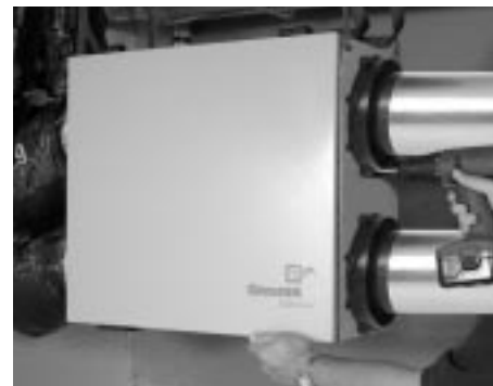
figure 6.6 Fix and secure with four screws supplied.
