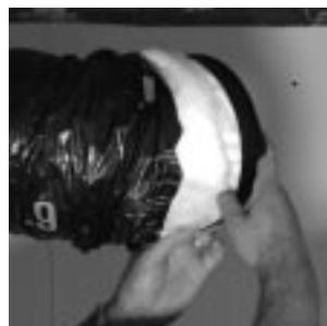
figure 6.3 Insert insulation inside the collar.
