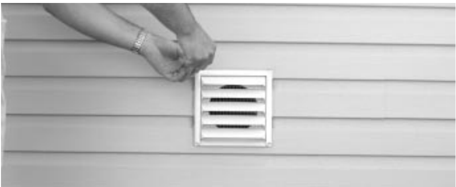
figure 10.4 Install Outside Hoods
