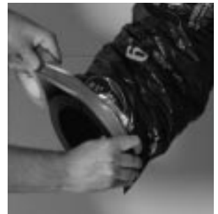
figure 10.4 Finish by taping the duct on the collar.
