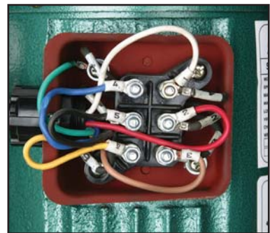
Figure 49. Motor wiring.
