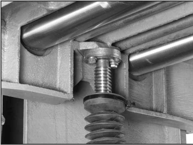
Figure 14. Column adjustment flange underneath table.
