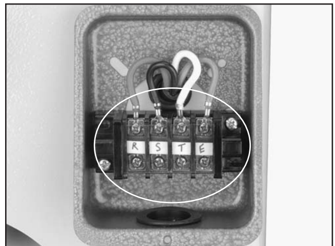
Figure 28. Main terminal located inside the electrical wiring box, on the outside of the cabinet.
