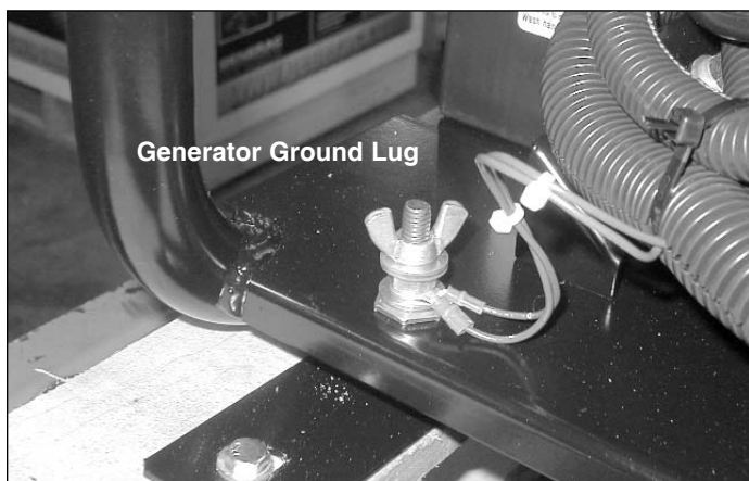
Figure 13 - Grounding the Generator
