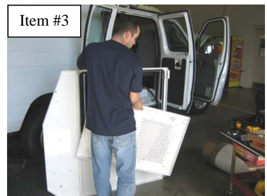
Remove Emergency Exit Hatch from Front Bulkhead to ease installation
