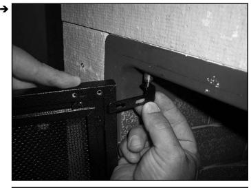
**Note:** The top hinges will mount to the door the same way as bottom hinges are mounted.
