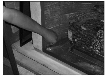
4. Remove the two screws in the top of left door.
