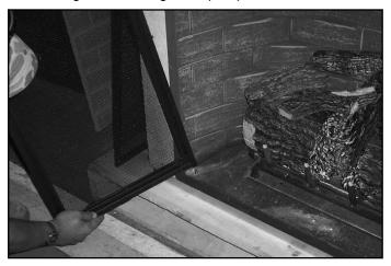
6. Insert door pin into hole of hinge pin provided in fastener pack and put into hole in upper left firebox top. Push pin up into hole to allow pin to fit on top of door.
