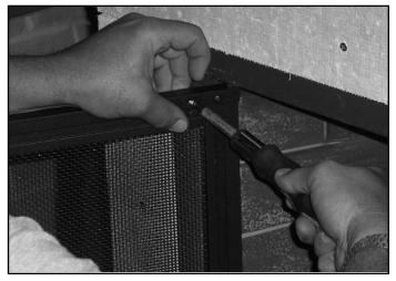
8. Attach door latch. Align the two holes in the door latch with the two predrilled holes in the bottom center firebox. Attach with the two screws provided in fastener pack.
