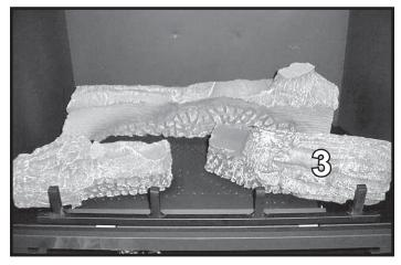
**LOG #3 (SRV327-703):** Position log #3 by locating its slot over the tab on the right front of the burner. The slot on the right side of log #3 fits over the bar grate.
