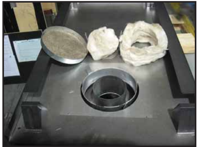
Figure 9.4 Remove and discard the seal cap, insulation donut, insulation plug, and the insulation basket. Attach the first vent section (it will snap into place). Slide the vent gasket onto the vent section and then, up against the appliance. Secure the vent gasket to the appliance with two self-tapping screws found in the manual bag. Note: The vent gasket can found in the manual bag.
