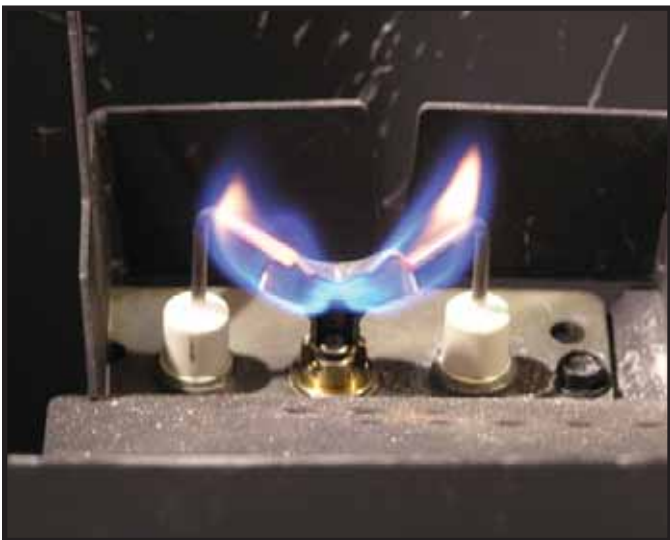
Figure 3.4 IPI Pilot Flame Patterns
