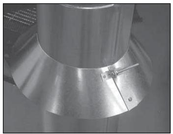
Figure 10.14 Assembling the Storm Collar Around the Pipe
