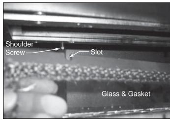
Figure 3.5 Reinstall Glass Frame
