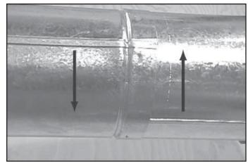
Figure 10.9 Rotate Seams for Disassembly
