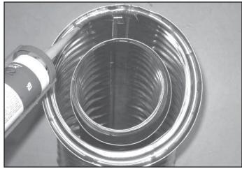
Figure 10.1 High Temperature Silicone Sealant
