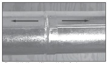
Figure 10.10 Align and Disassemble Vent Sections
