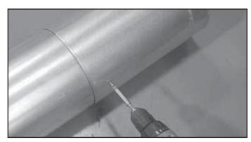
Figure 10.6 Screws into Slip Section
