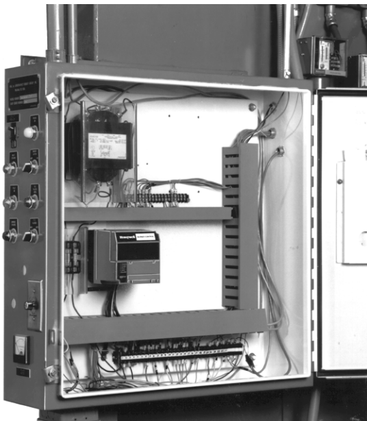
Fig. 7. Electrical panel installation.
