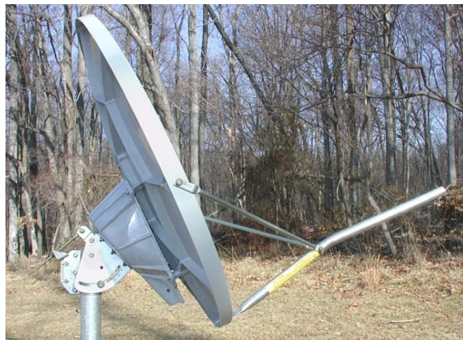
Figure 22: Completed antenna assembly (without radio)
