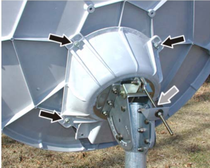
Reflector attached to bracket
