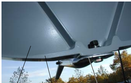
Back of reflector Rim Flat end of feed support tube
