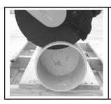
Rotate Pipe and repeat this cutting process until pipe circumference is cut.
