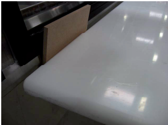
Step 7: Mount wrap board on top of bracket using a 1/4" spacer to have a gap between rear wall and board.
