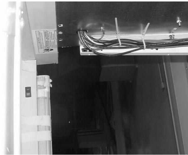
RLT Wiring Routed Up Through Top Panel to Wireway on Top
