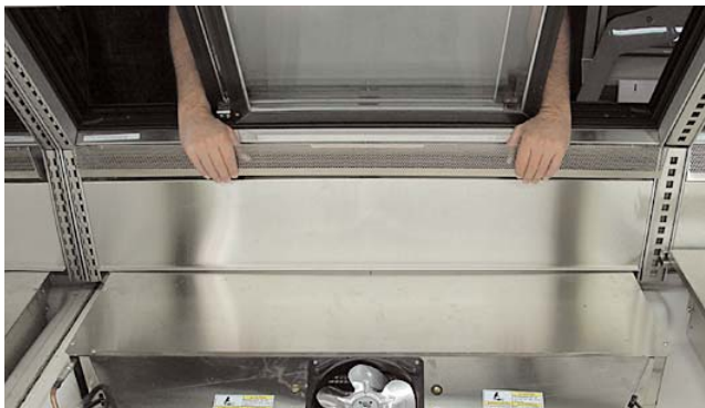
STEP 7 – Lift out discharge air grille.
