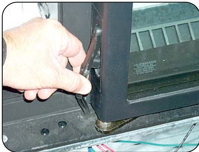
Figure 5. Removing the Heater Terminal Plug
