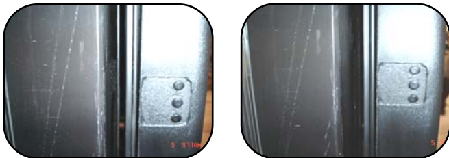
Before and After Gasket Conditioning
