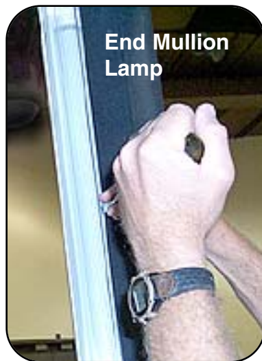
Figure 21. Removing Diffuser from End Mullion Lamp
